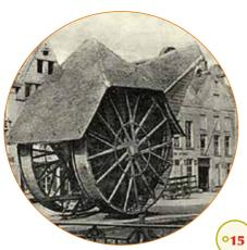
Crane bridge?! Exactly! Six hundred years ago, there was an enormous crane just past the house The Little Devils, on the other side of the bridge, which would unload and load the ships that docked here. In order to operate the crane, people had to walk in the giant wheels of the crane! Those people were called the crane children.
